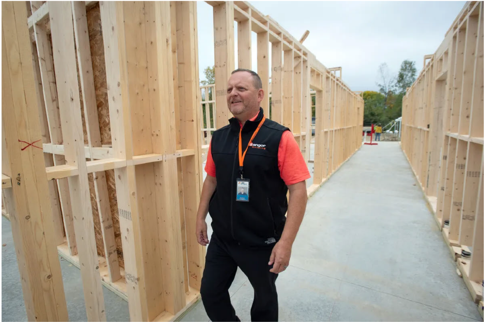
Michael Myatt, executive director of BangorHousing, walks through the new construction of Sunridge Senior Housing, a 50-unit senior living complex on Sunset Avenue in Bangor, in September 2025. Credit: Linda Coan O'Kresik / BDN
